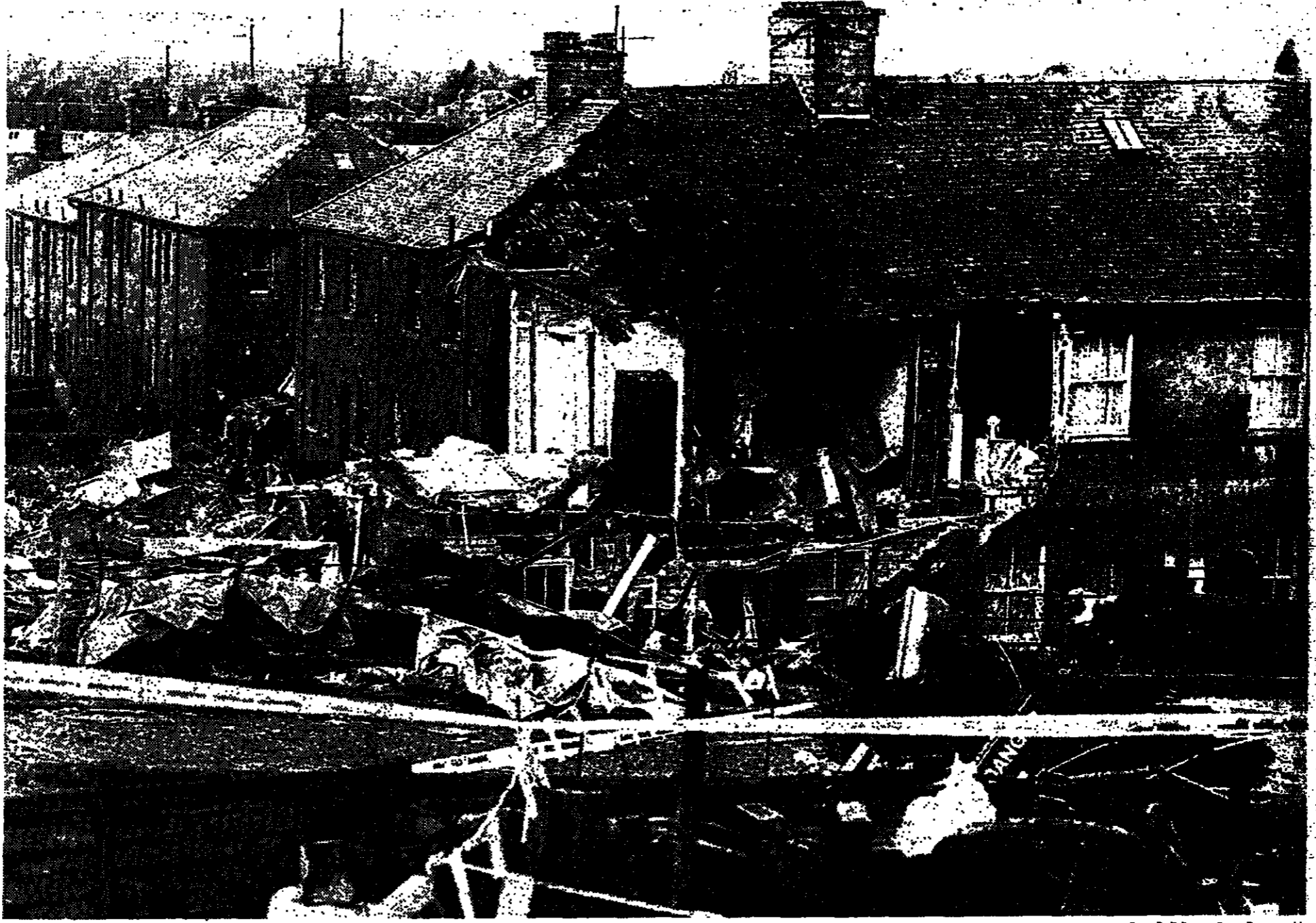
A wardrobe stands undisturbed amid the devastation of Lockerbie. The wreckage of these houses spilled on to the A74 and into the gardens of neighbouring homes.
